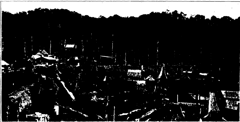
Fig. 3. National Coal Company's plant at Butong.
